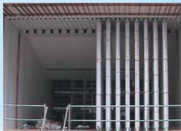
中・低周波数用200mm厚 吸音スプリッタ Medium/low-frequency noise absorption splitter (200mm thickness)
